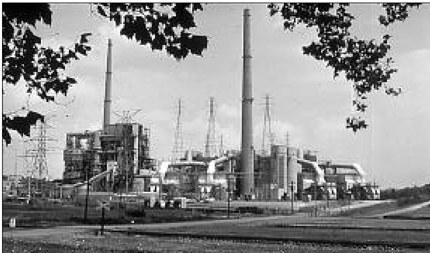
Coal-fired power plant with electrostatic precipitators visible. Photo courtesy of American Electric Power.
