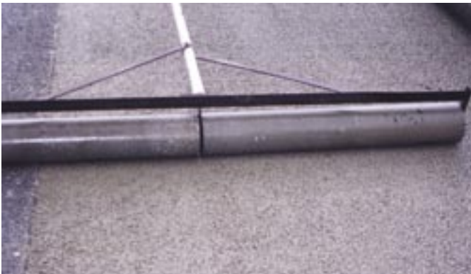
Fig. 3: Pervious concrete should be cross-rolled when fresh to smooth it out
