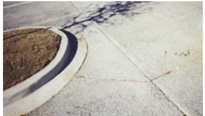
Fig. 5: Rules about jointing are the same with pervious concrete as with any concrete
