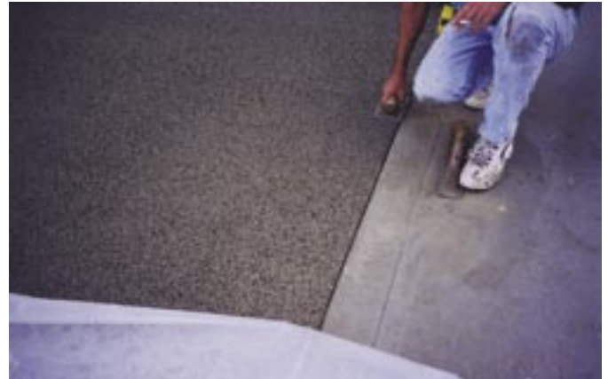
Fig. 4: The owner may prefer the look of a rounded edge adjacent to a sidewalk
