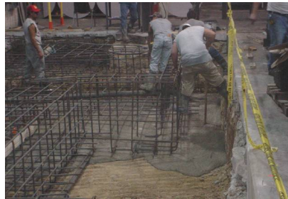
Moving the hose around all the steel
