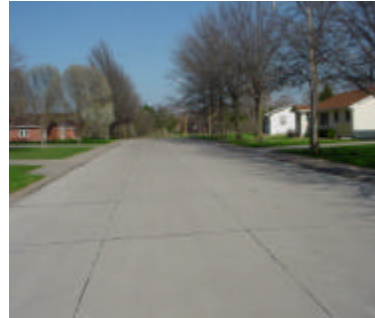
With Concrete streets
